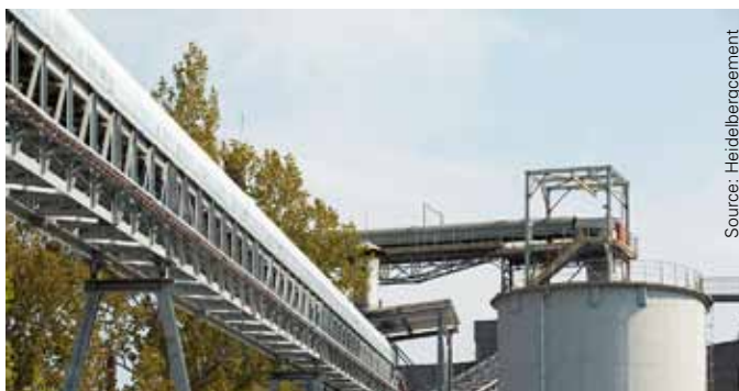
At the Carpatcement plant in Deva, limestone is transported from the quarry to the manufacturing plant by long conveyors
