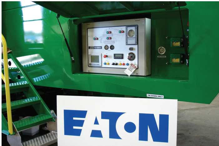
The screen on the control panel "talks" to the EFX controllers.
