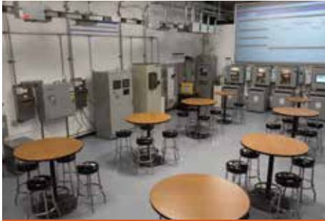
Power quality lab
