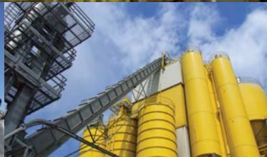
Kiln and refractory
