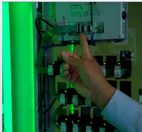
The flat cable plugs into the back of the HMI-PLC unit, eliminating a gateway or communication card. It connects serially to other control panel devices using a snap-in connector for each. Courtesy: CFE Media
