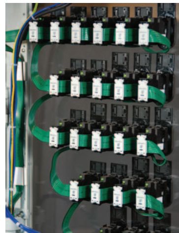
Figure 6. Device-level wiring systems use flat multiconductor cables to connect components, replacing bulky wiring ducts found in conventionally wired control panels.
