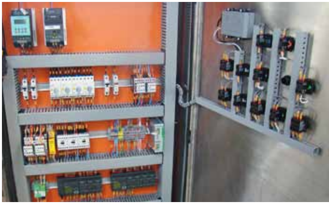
Conventional control wiring
