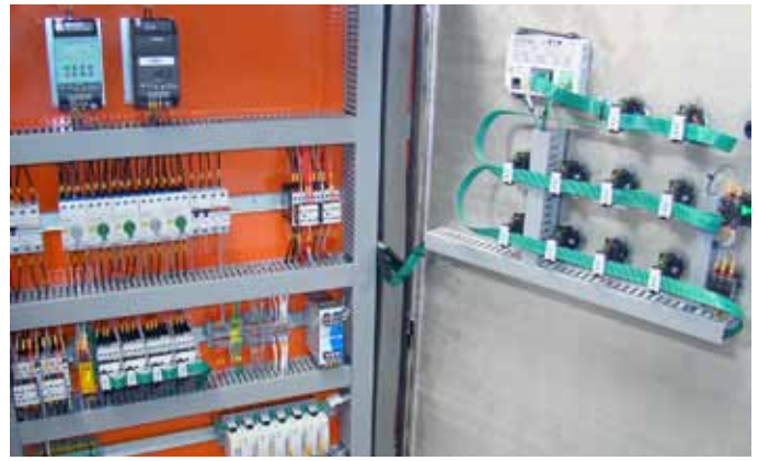
Lean Solution with HMI/PLC and SmartWire-DT: The wiring time was reduced by 94% and data transparency considerably increased
