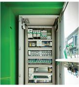
Eaton's PKE and PKZ manual motor starters and DIL contactors have been tried and tested for both IE2 and IE3 motors
