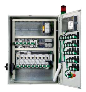
Figure 5. Control Cabinet After a Device-Level Network like Eaton's SmartWire-DT<sup>®</sup> System Connects Devices, While Eliminating the Hassles of Traditional I/O Wiring.
