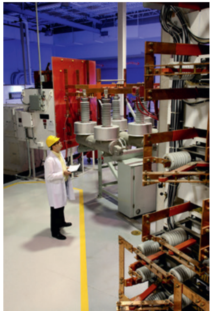
The Eaton Bussmann Division's Paul P. Gubany Center for High Power Technology is the electrical industry's most comprehensive facility for testing and certifying device and equipment SCCRs. Capable of performing electrical tests up to 600 volt three-phase, 300,000 amps of short-circuit current for meeting ANCE, ANSI, CE, CSA, ETL, IEC and UL testing requirements.
