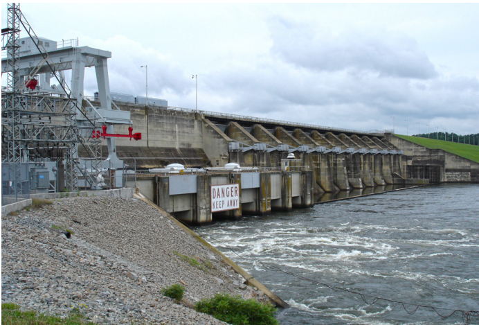
Figure 4. Gaston Hydro Station
