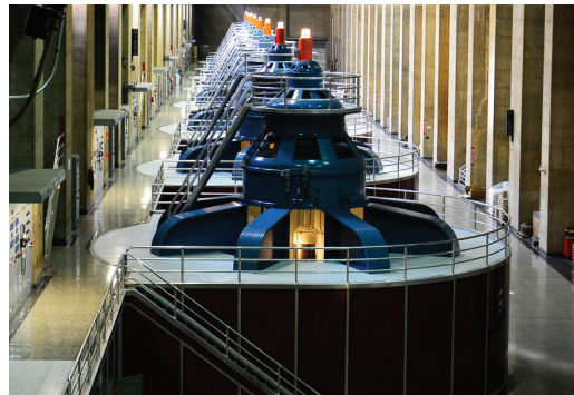
Figure 1. Typical Hydro Generators
