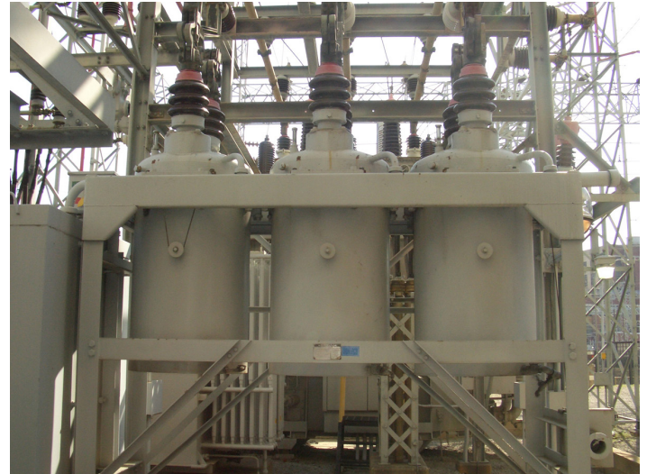
Figure 5. Typical Oil Circuit Breaker
