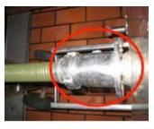
Fig. 8: Incorrect, unsuitable extension piece
