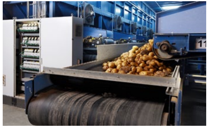
Intelligent bunker filling: Laser sensors control the conveyor belts and ensure an even transport volume.
