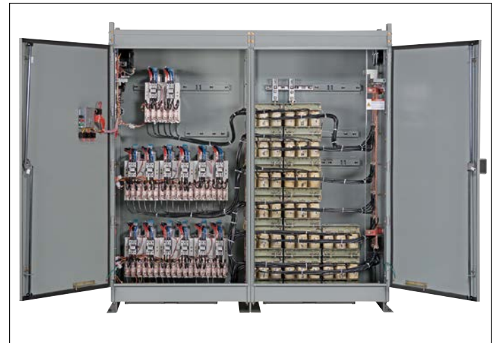
Figure 15. Switched harmonic filter [16]
