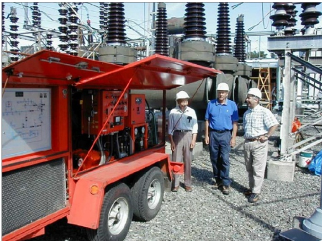
Fig. 4: Image of a standard gas cart used for inspection and repair of SF6 utility assets.
