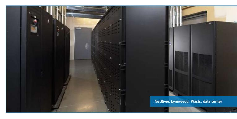
In addition to the UPSs, NetRiver complemented its overall power protection solution with three Eaton Power Distribution Units (PDUs) and five Eaton Rack Power Panels (RPPs) — dual-fed quad panels that bring high-density power distribution closer to IT enclosures to streamline cabling while providing a more adaptable infrastructure.
