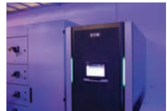
The Eaton 93PM 120 kW UPS guarantees power supply for a defined period to critical loads in the event of a power failure.
