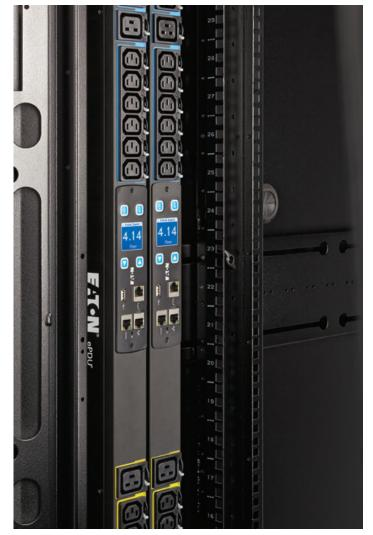
Figure 1. Rack PDUs with racks from the same vendor ensure compatibility, which enables agility in the data center.
