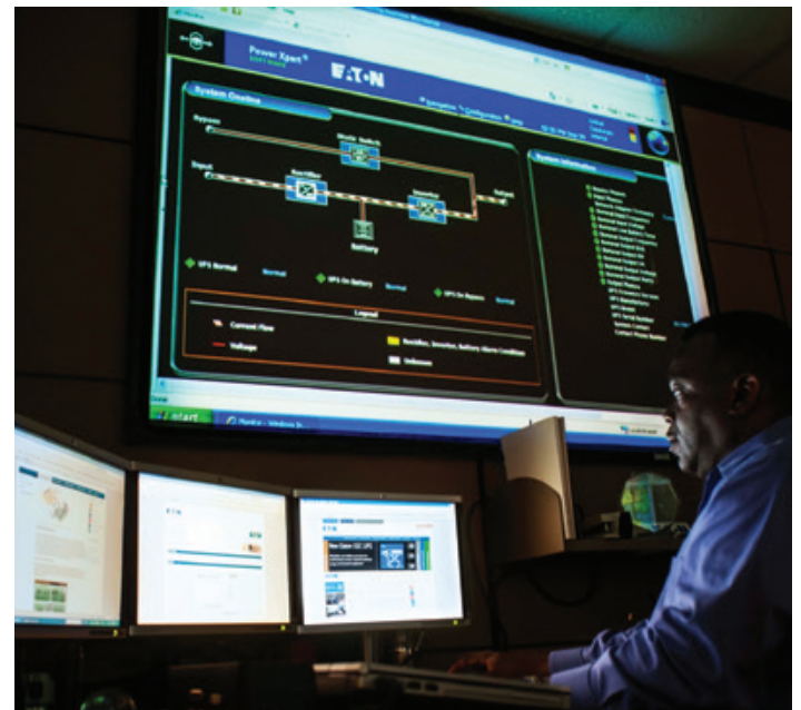
With the service upgrades, MWO received eNotify, which makes it easier to monitor the UPS from the valley and from our monitoring center in Raleigh, NC.
