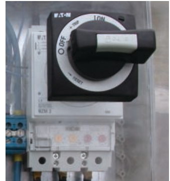
Kemper has installed Eaton's NZMN2-VE250 circuit breaker in a prominent position on the dashboard. In this image, it is combined with a turning handle to switch it on and off (source: Kemper)
