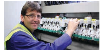
With the use of SmartWire-DT, all motor protection switches become smart and communication-enabled components; Claus Buhrmester, BASF: "We can distinguish whether it is a runtime error due to an overcurrent or frequent switching on and off."
