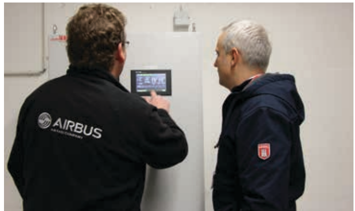
Eaton's BreakerVisu collects all data from the circuit breakers, from the diagnostic system for temperature measurement and from the Arcon arc fault protection system, and communicates via Modbus directly with the building management system
