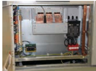
The Arcon arc fault protection system increases personal safety
