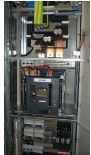
Eaton's IZM circuit breakers, which are fitted with an electronic trip unit and integrated measuring function, are used
