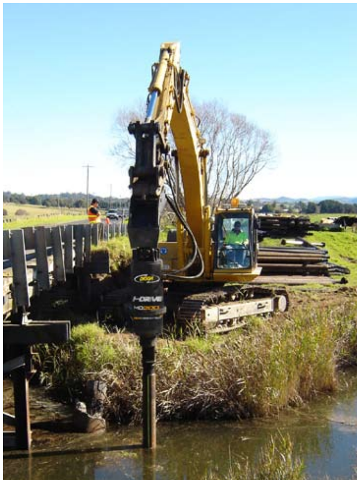
Attached to the boom of an excavator, the I-Drive is used for tasks including core barreling, screw anchoring, and foundation drilling. The compact I-Drive allows these operations to be performed in confined areas and close to existing structures.
