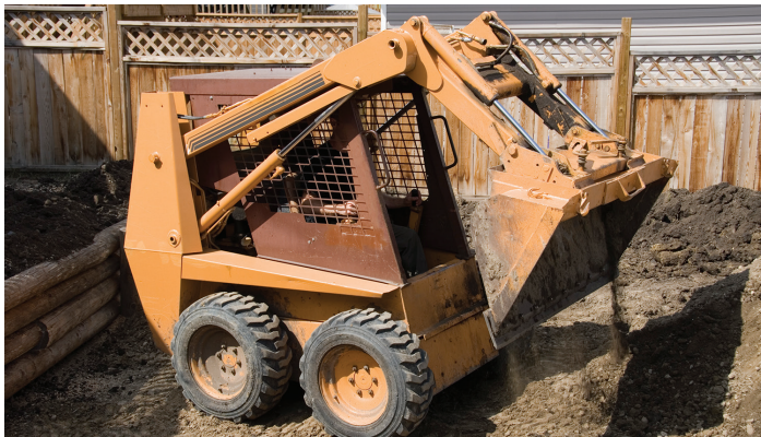
Skid steer loader working in tight conditions
