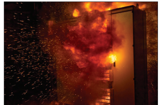
Figure 1. An arc flash can ignite large and dangerous explosions.
