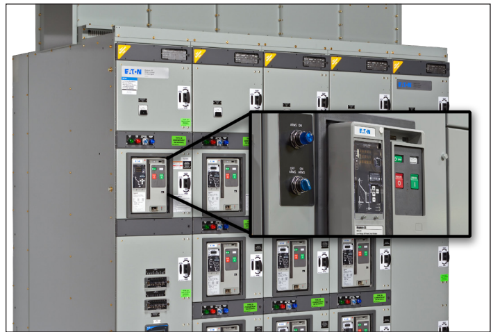
Figure 3. An Arc Flash Reduction Maintenance System shortens fault clearing times by bypassing time delays in the trip circuit.
